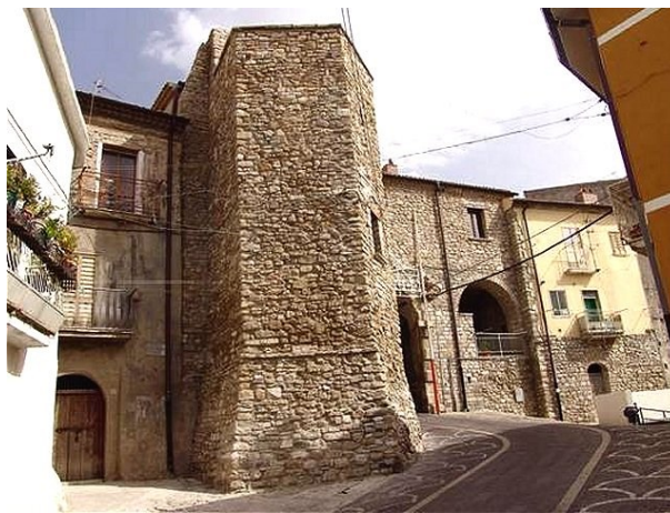
Figure 1. Medieval Town Walls of Tolve
